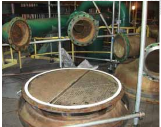
GORE® Series 300 Gasket Tape installed on an evaporation condenser.
